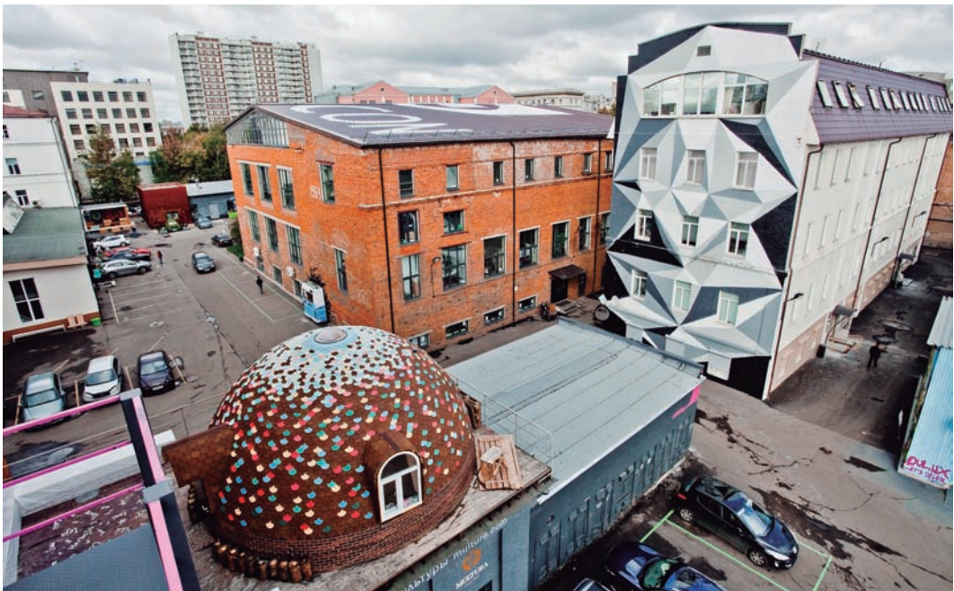
Photographs courtesy of Facon Design Factory
